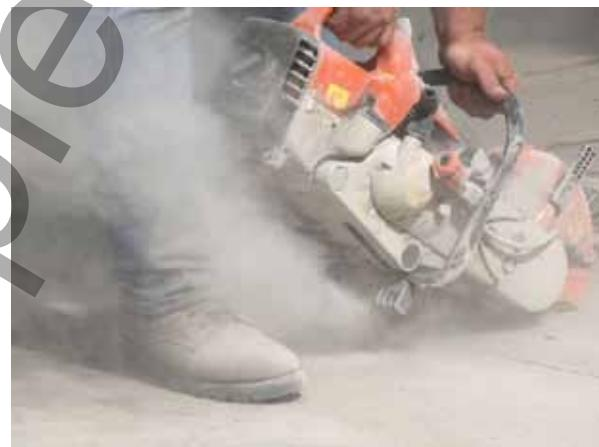
*Cutting concrete creates high levels of cement and silica dust*
